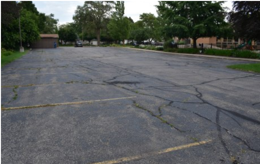
Before, during and after photos of the parking lot project!
